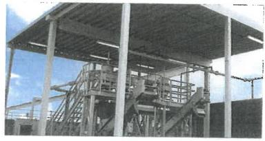
aerated grit chambers provided significant savings, not only in capital investment, but also in annual operation and maintenance cost and overall life-cycle cost. Other improvements included structural repairs around anchored slide gates, replacements of the gates and addition of electrical actuators.
